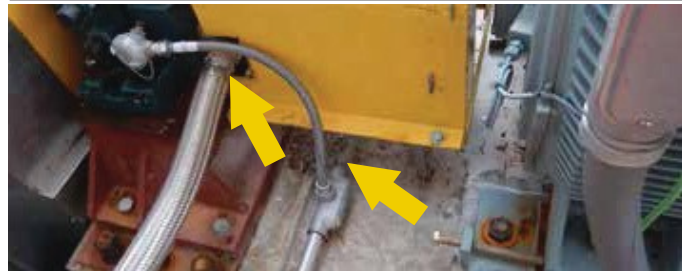
EXAMPLES OF OBSTRUCTIONS THAT WE WOULD NEED TO KNOW ABOUT
