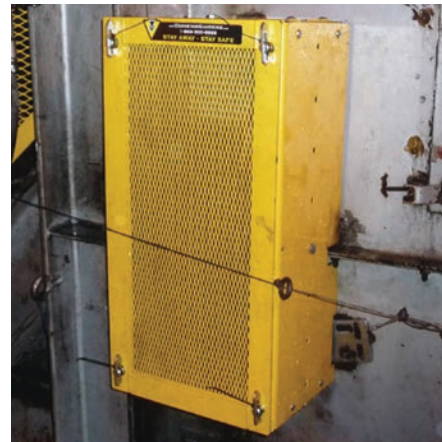
3 Guard installed over exposed bearing
